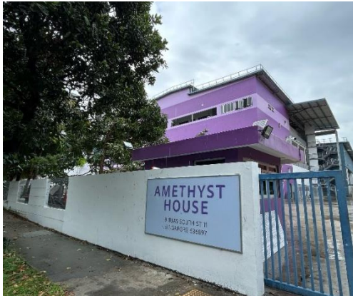
Amethyst House — 9 Tuas South Street 11
